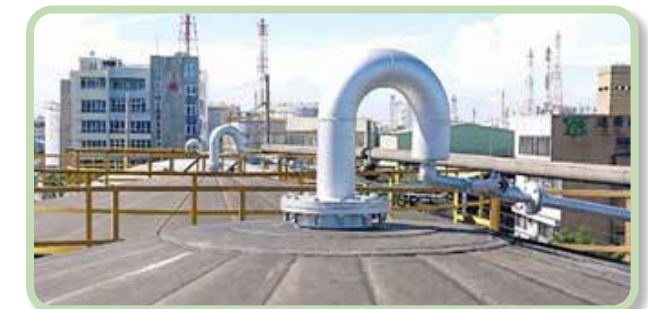
Breather valve connecting pipe setup
